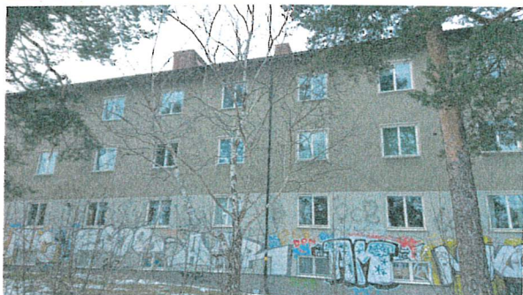
baksida bef. fasad
