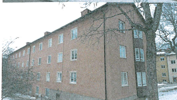
baksida bef. fasad
