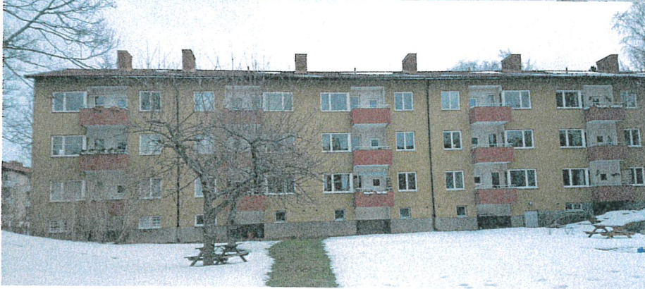
baksida bef. fasad
