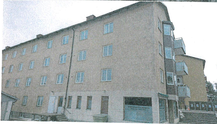
baksida bef. fasad
