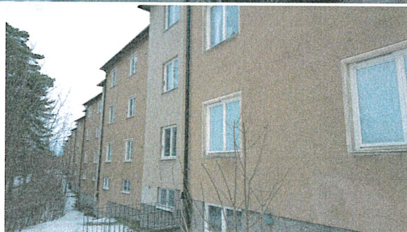
baksida bef. fasad
